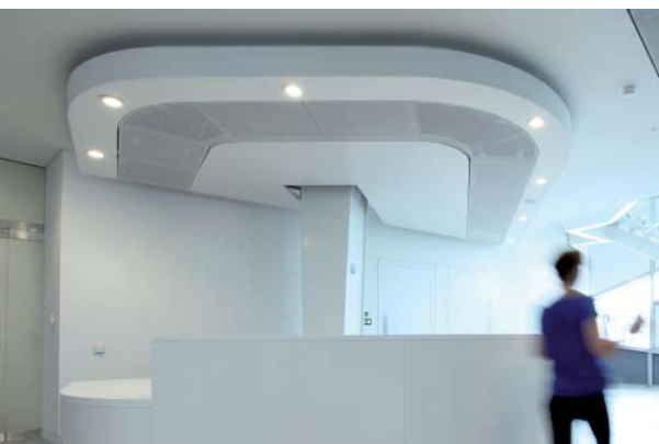
DALI LED lighting was controlled by KNX
